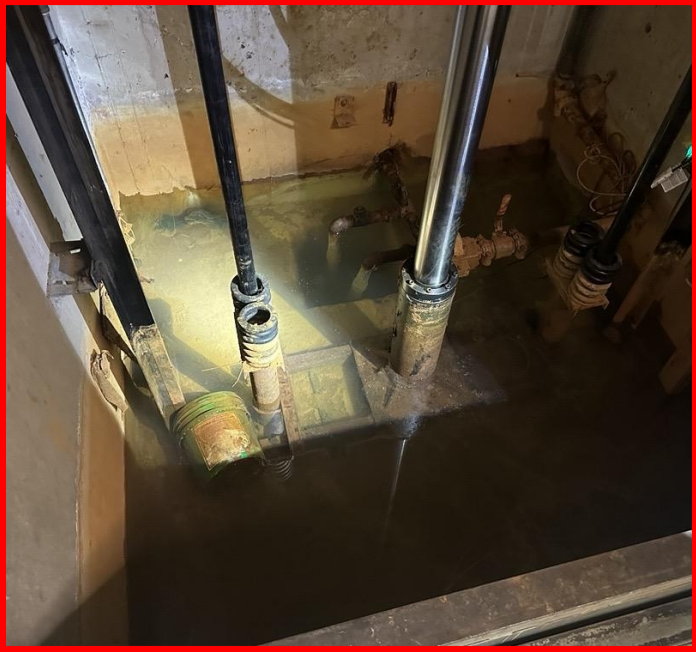
Freight elevator pit
