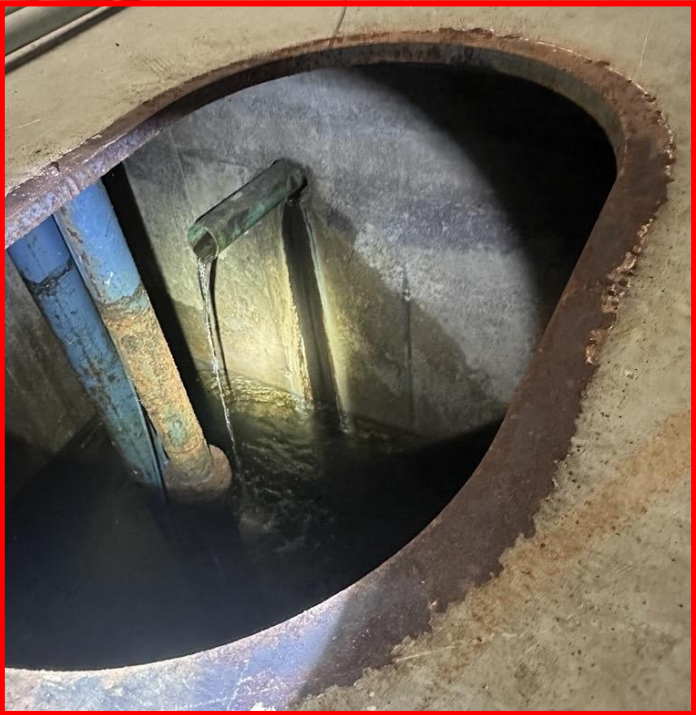
Constantly draining into sump room
