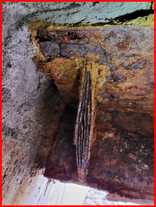
Beam to foundation wall connection at underside of bridge
